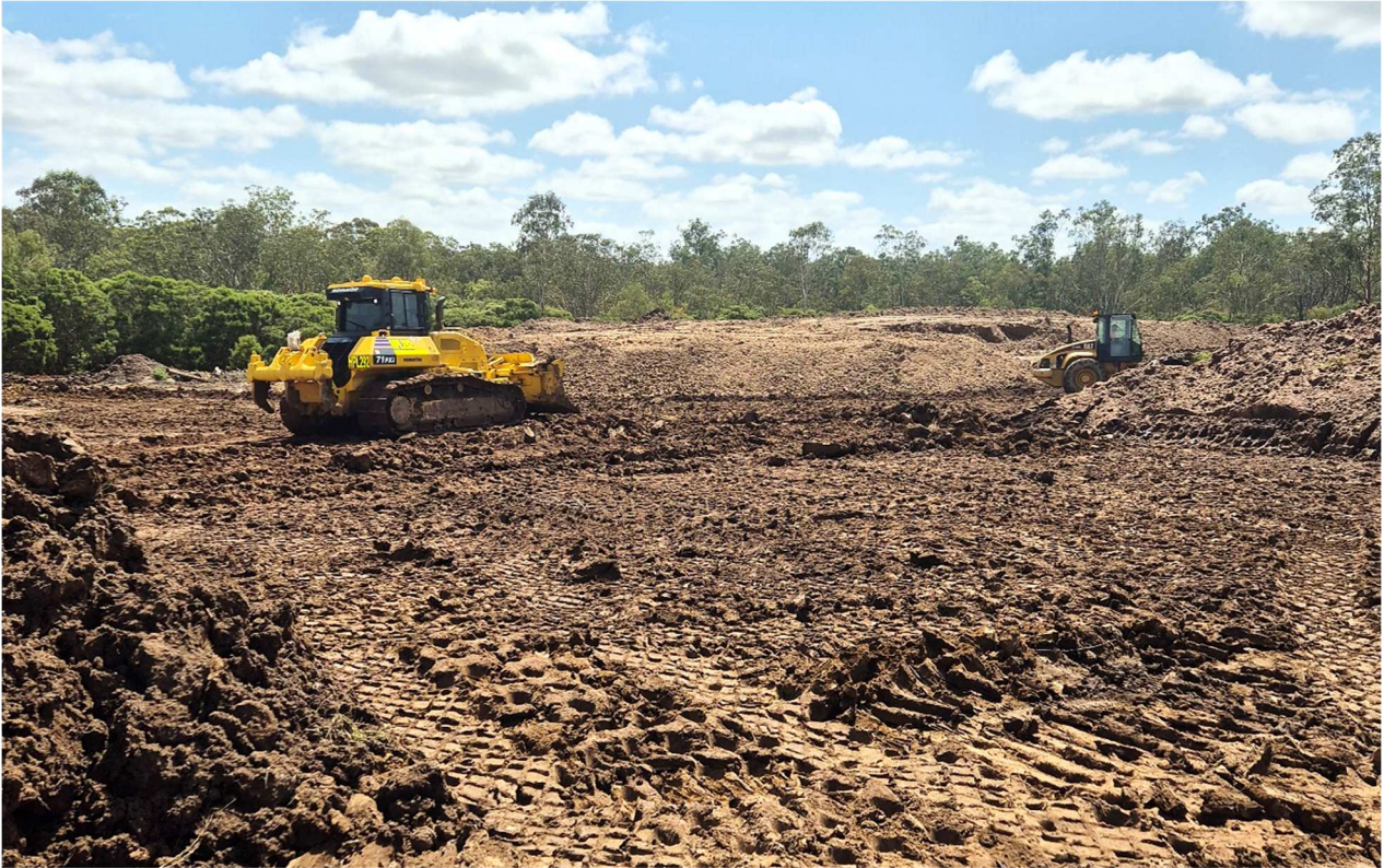
Figure 3: Proof rolling operations in progress – (12/12/2024)
