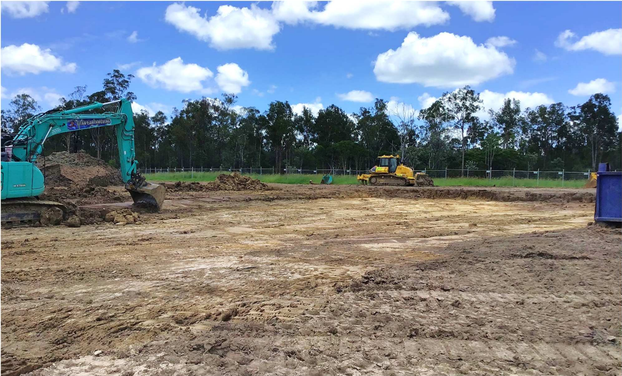
Figure 5: Strip filling operations in progress – (13/12/2024)
